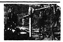
Field maintenance was simple in the shallow settings used in Tanzania, because the complete pumphead, together with rising main and pumprods, could be pulled out in one piece. Nevertheless, a substantial tool kit is required, and at greater depths (beyond about 6-8 meters) the pump is more difficult to maintain.
