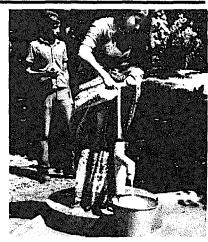
essential interventions were mainly to replace footvalve parts (O-rings and body) or leather cupseals. Sand entry into the well is a problem in Bangladesh, and leather cupseals are not suitable in these conditions; nitrile rubber seals have proved substantially better.
