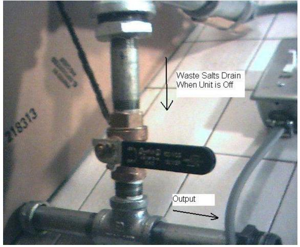
This upside down "T" has two purposes. It helps hold the unit up and it allows salts to be drain off when the unit is turned off. Neither one are essential to operation. The unit designed for open fire use has a clean out plug at this point. The salts tend to deposit on the walls of the boiler tube with time. Frequency of cleaning will depend on the hardness of the water source.
