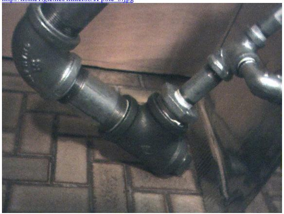
Notice the 1.5 inch clean out pipe plug on the right bottom. This is to be used to clean out the salts that accumulate at regular intervals. The time frame will depend on the hardness of the input water.
